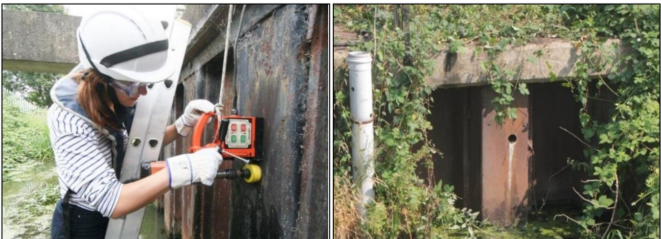
Kingfisher nesting hole incorporated into the sheet piles at the Board's Pumping Stations
